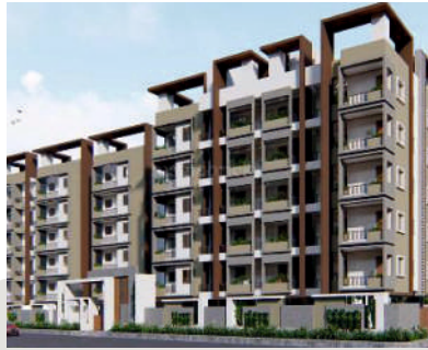
NMR Group (Thurkamjaya)
